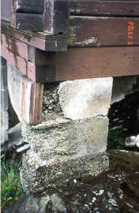
Figure 2: White Sulphur Springs Bathhouse Foundation Showing Crumbling Concrete
